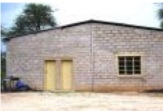
Two Store Rooms
