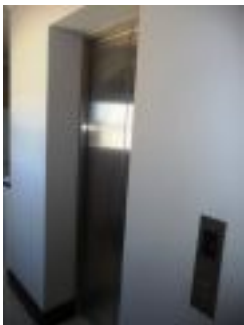
Lift to Penthouse
